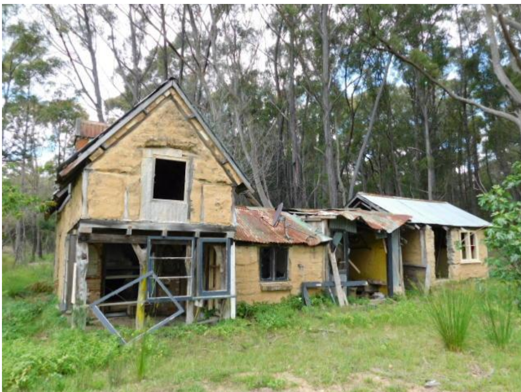
Above: Building 2 going from west to east on the site called The Magic House . Consists of three sections all of mud brick. Three sections built at different times so method changed/advanced.
