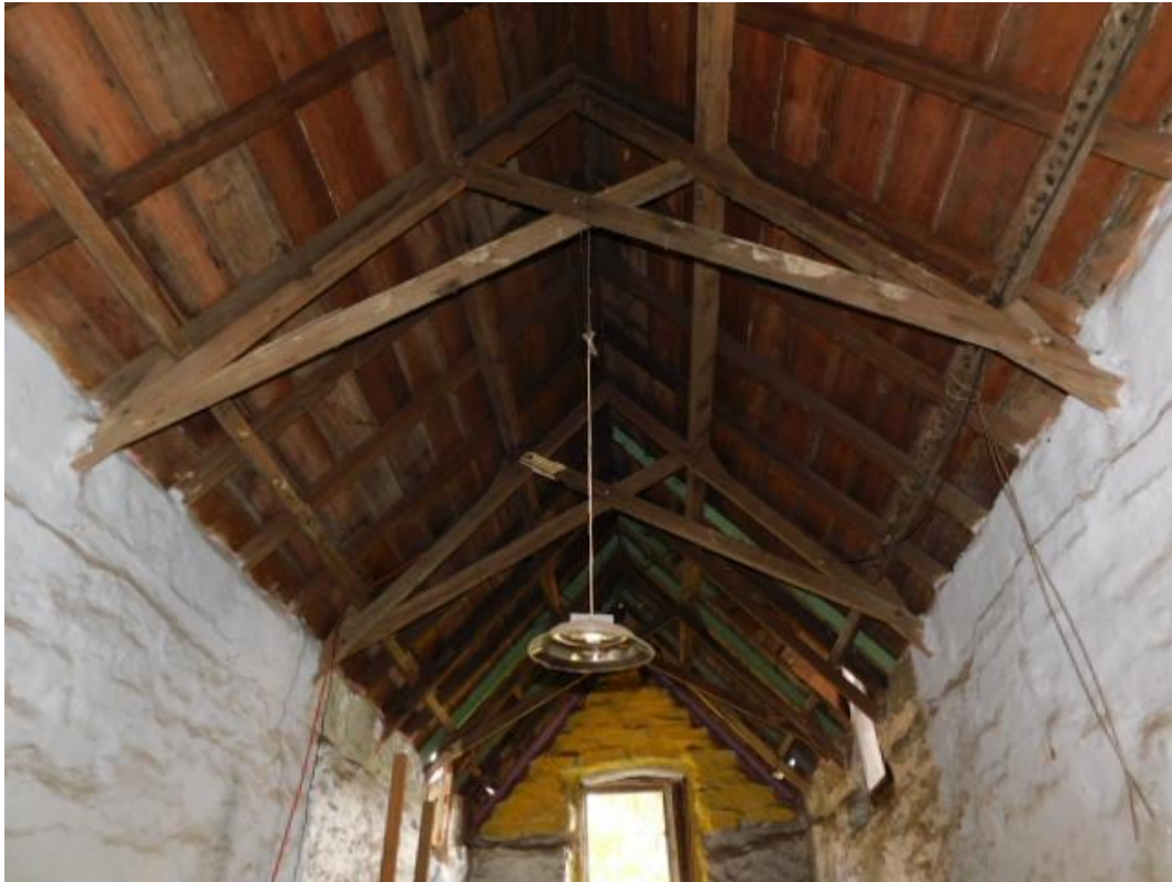
Above: interior of Building 2 The Magic House showing milled roof frame and lining boards.
