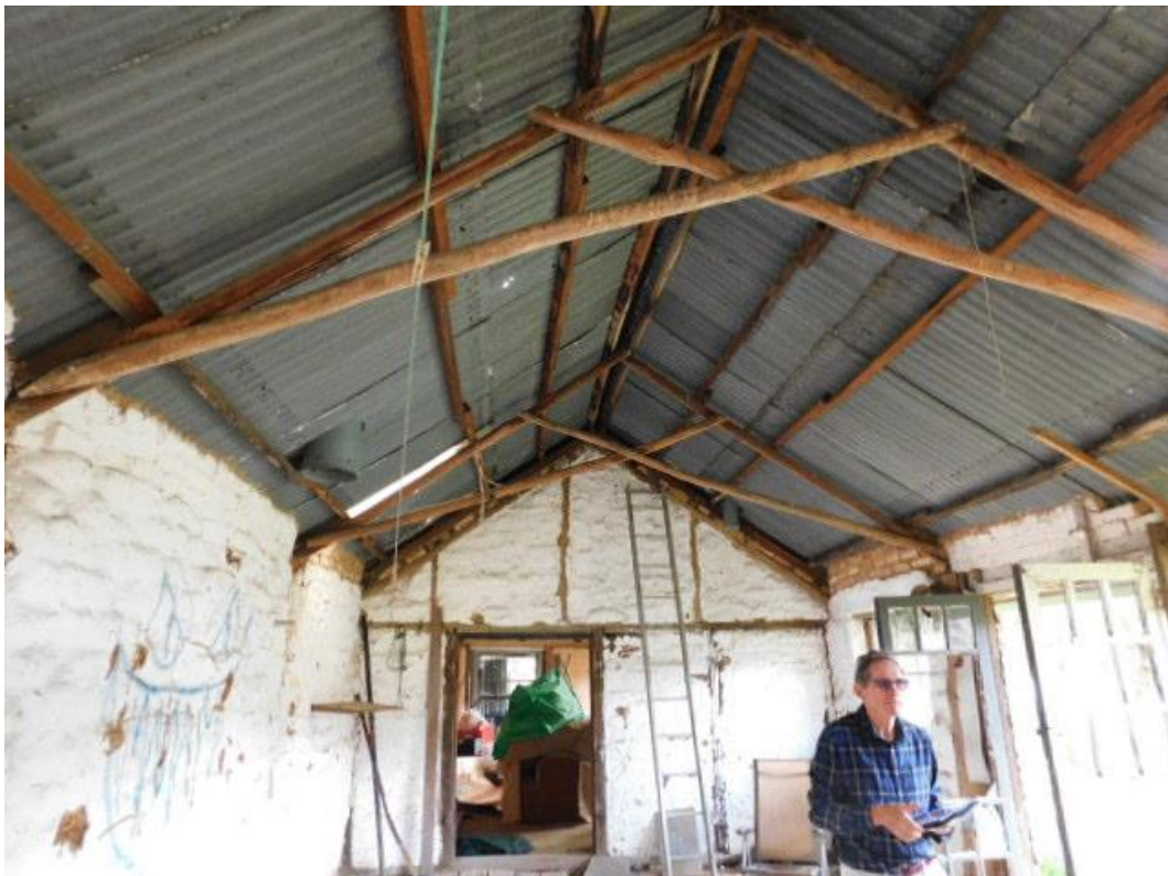
Above: Interior of Building 1 The Studio showing round pole roof frame. Mark Williamson's comments on this photo by email on 14/1/2022 Both the 2 scissor and 2 king post/half scissor trusses use local stringy bark.
