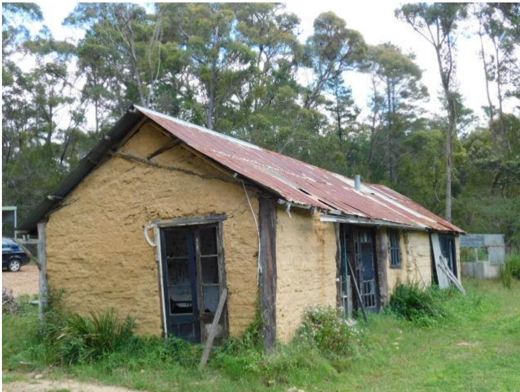
Above: Building 1 going from west to east on the site called The Studio . The western (right) end is rammed earth. The eastern end is mud brick. Two sections built at different times so method changed/advanced.
