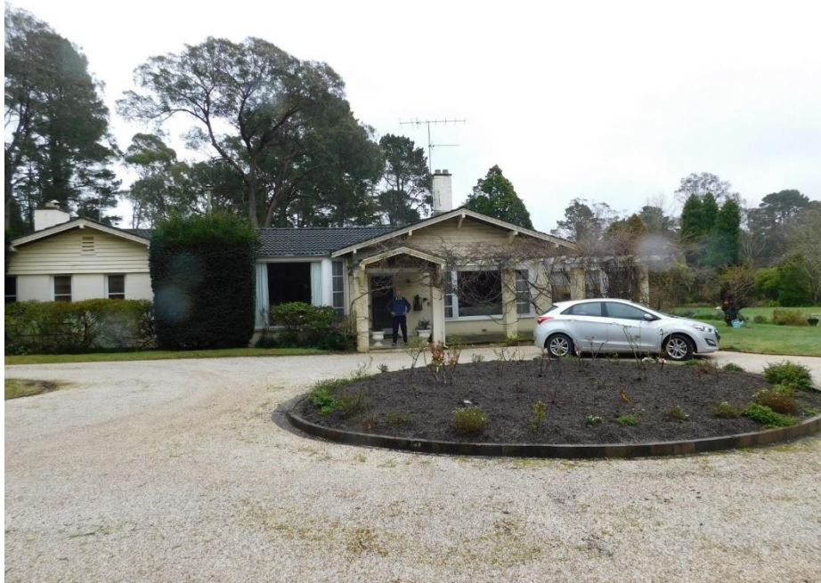
Above: Tregarthen, September 2022. Circular drive and eastern elevation showing low pitched roof with large exposed timber supported eaves. Gabled section to the left houses the Kitchen and chimney and the gabled section to the right houses the Living Room and chimney. Dining Room is located between the two.
